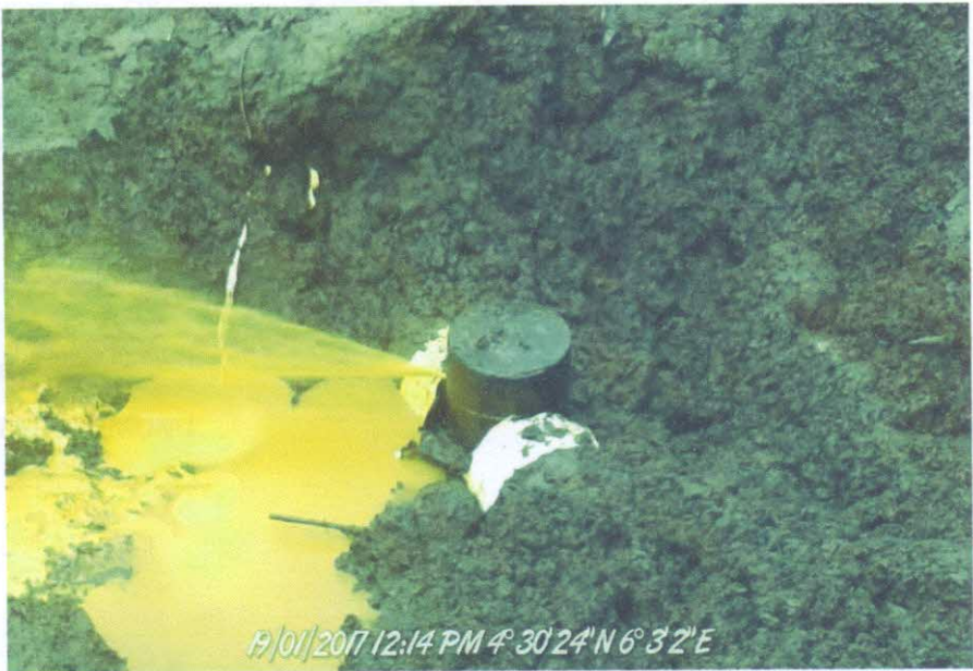
SPILL POINTS AFTER EXCAVATION SHOWN: fig3
