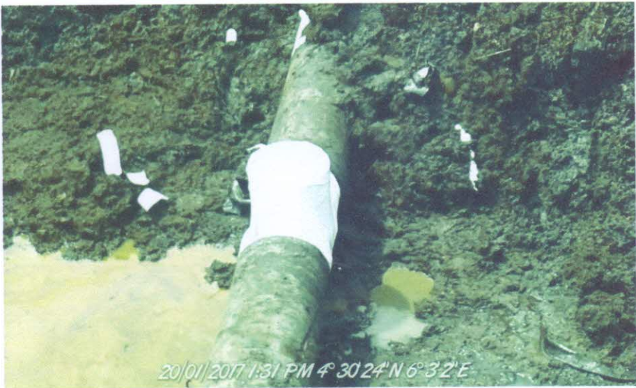
SPILL POINT AFTER REPAIRS: fig4
